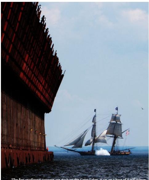
.... The first reinforced concrete ore dock on the Great Lakes, it sits on a base of 9,809 pilings of Oregon fir driven 20 feet into the lake bottom. A 9-ft, thick cap of reinforced concrete tops the pilings, making a foundation that has endured 100 years of vibration from train engines and ore cars.
