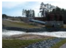
Remnants of the Tourist Park Dam.
